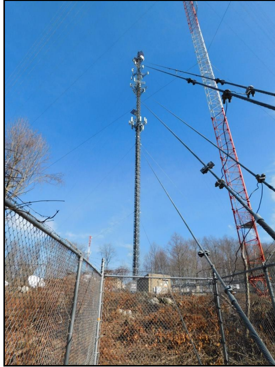
Photo 3 – View of new guy level 1 and 2 guy wires
