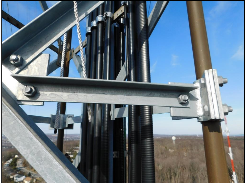
Photo 6 – New horizontal and diagonal sub-bracing installed on the tower
