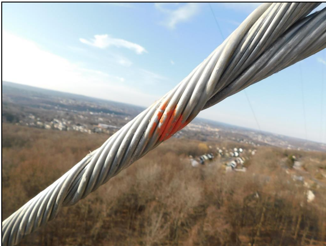
Photo 2B – Another view of new guy wire at the tower end
