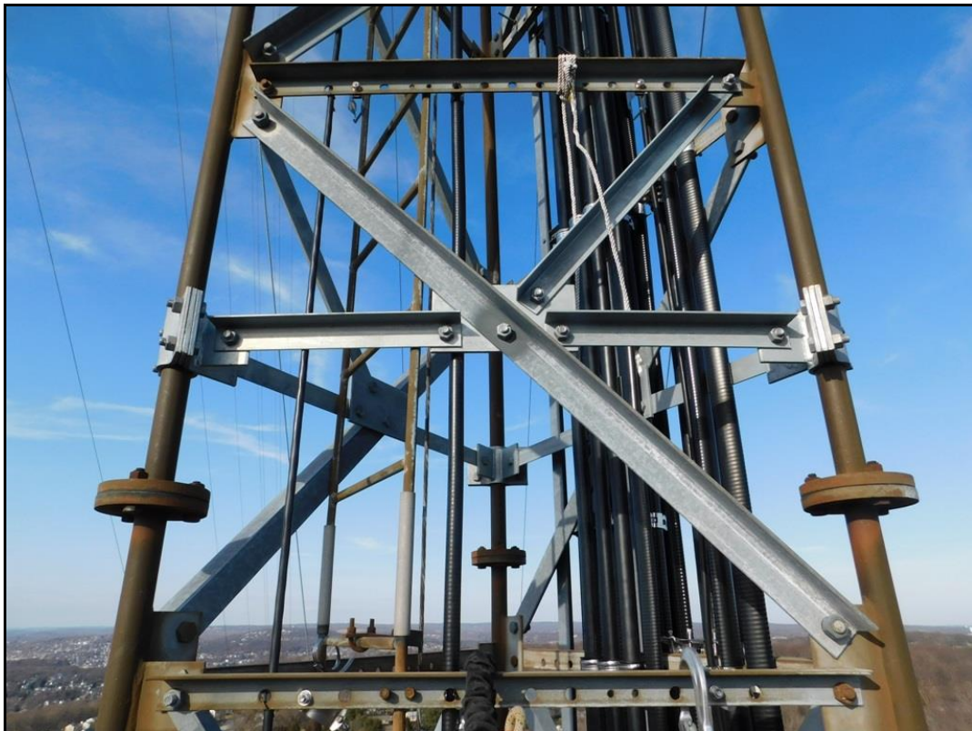
Photo 4 – New horizontal and diagonal sub-bracing installed on the tower
