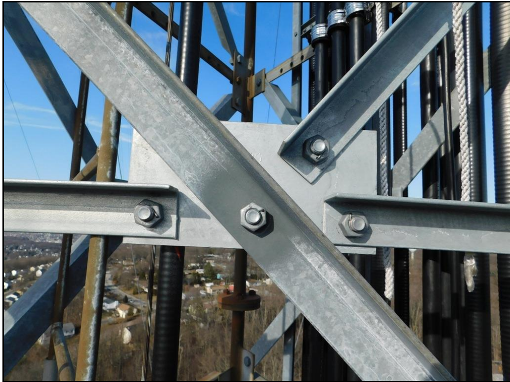
Photo 5 – New horizontal and diagonal sub-bracing installed on the tower
