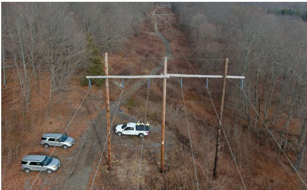
DCHF Structure without Cross or Knee Bracing
