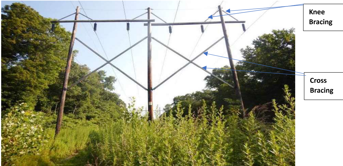
DCHF Structure with Cross and Knee Bracing
