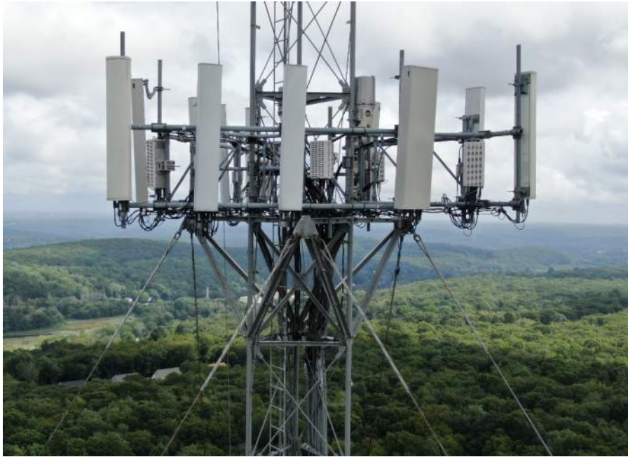
Photo 1: Photo illustrating the Tower with Appurtenances shown.
