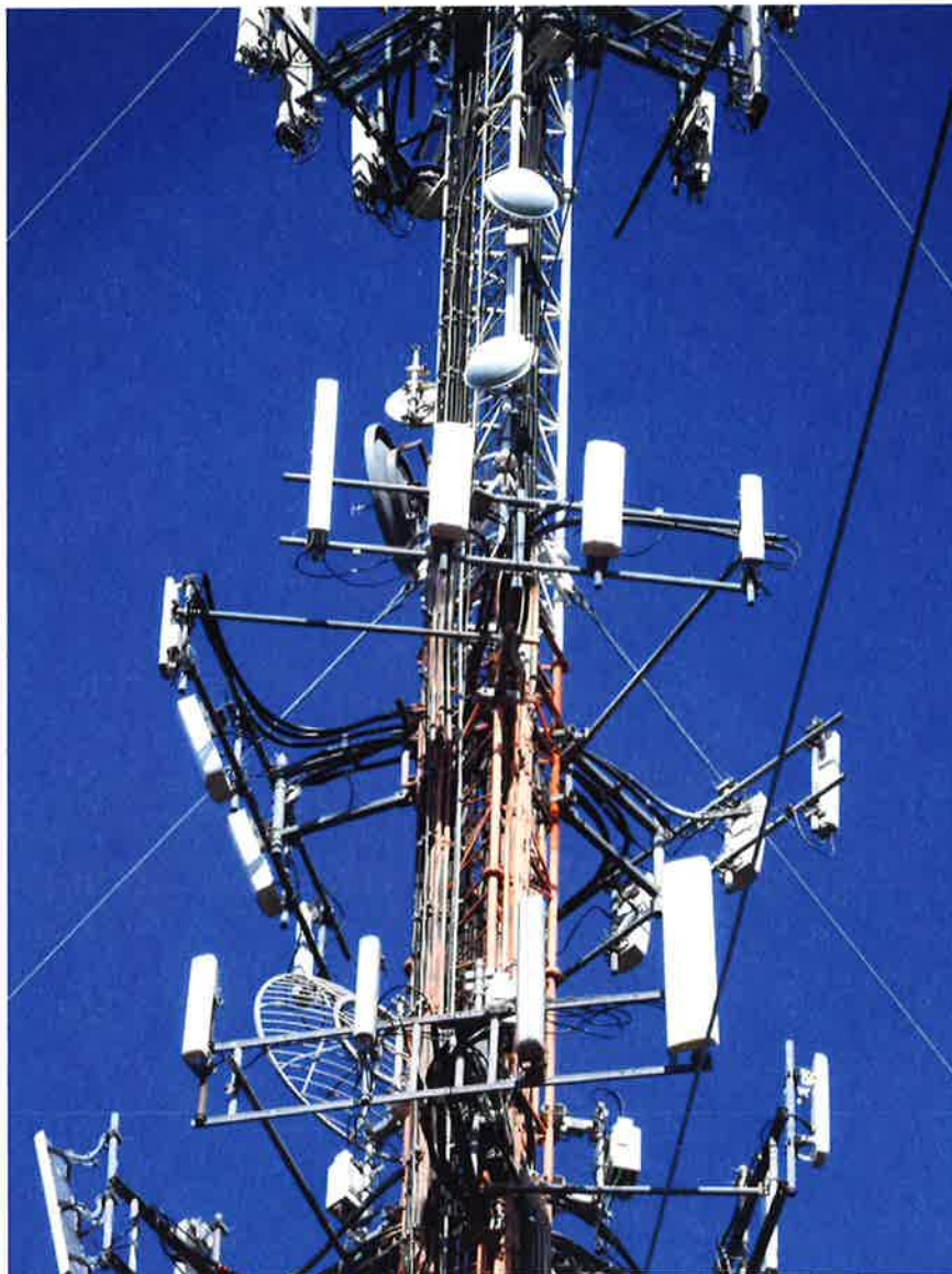
Photo 1: Photo illustrating the Tower with Appurtenances shown.
