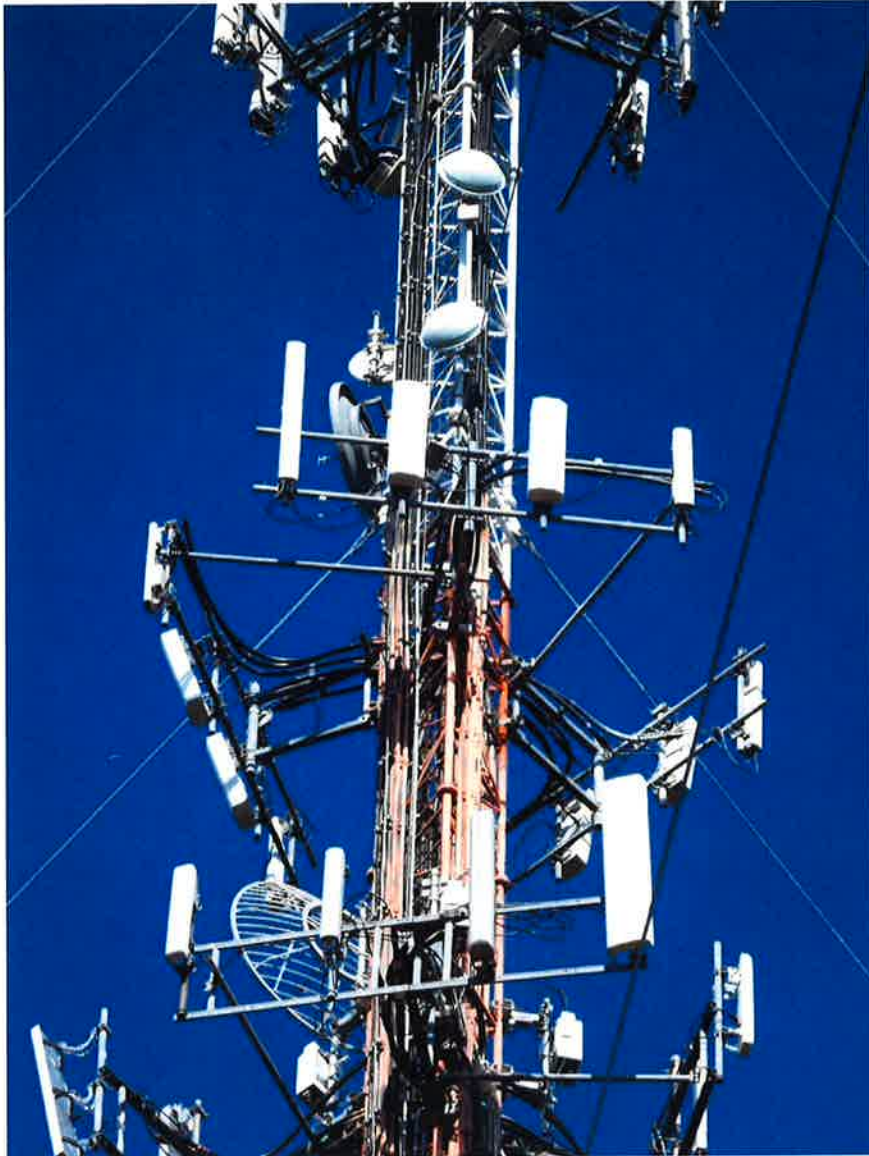
Photo 1: Photo illustrating the Tower with Appurtenances shown.
