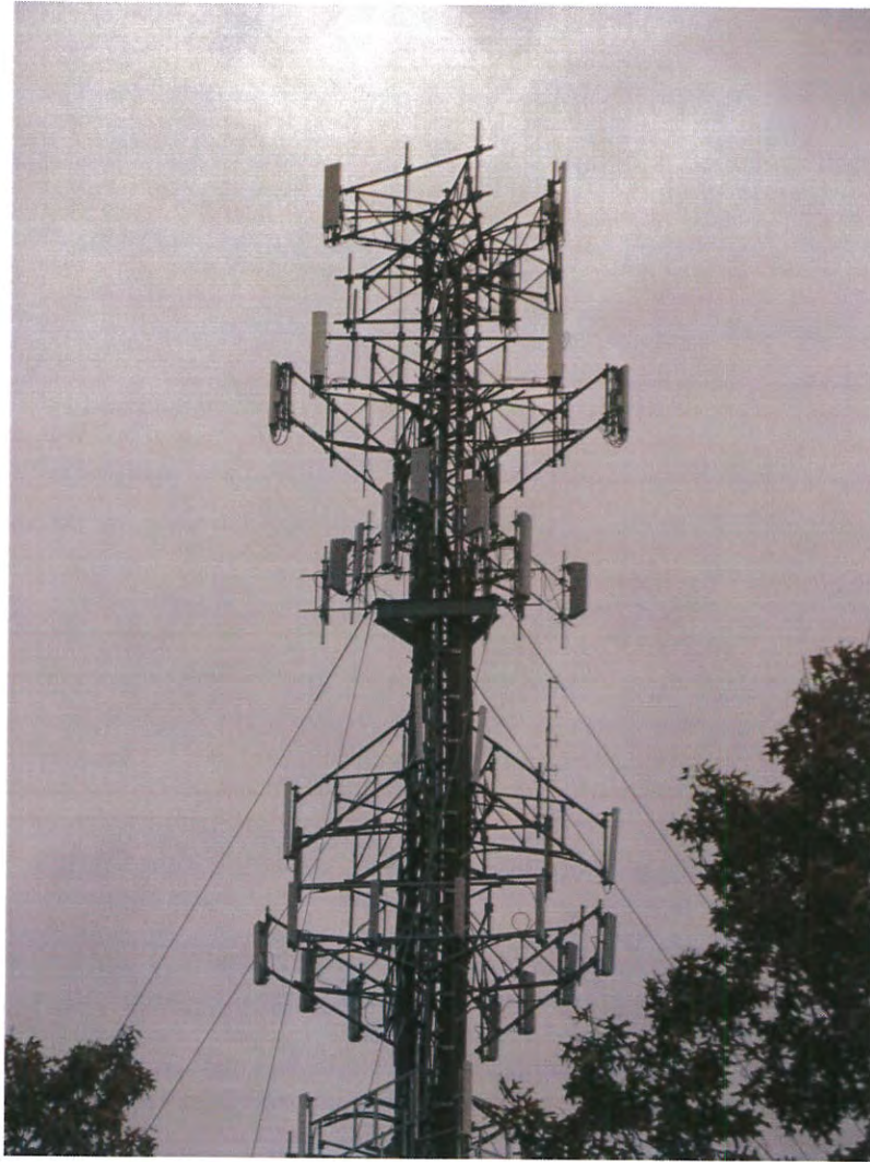
Photo 1: Photo illustrating the Tower with Appurtenances shown.
