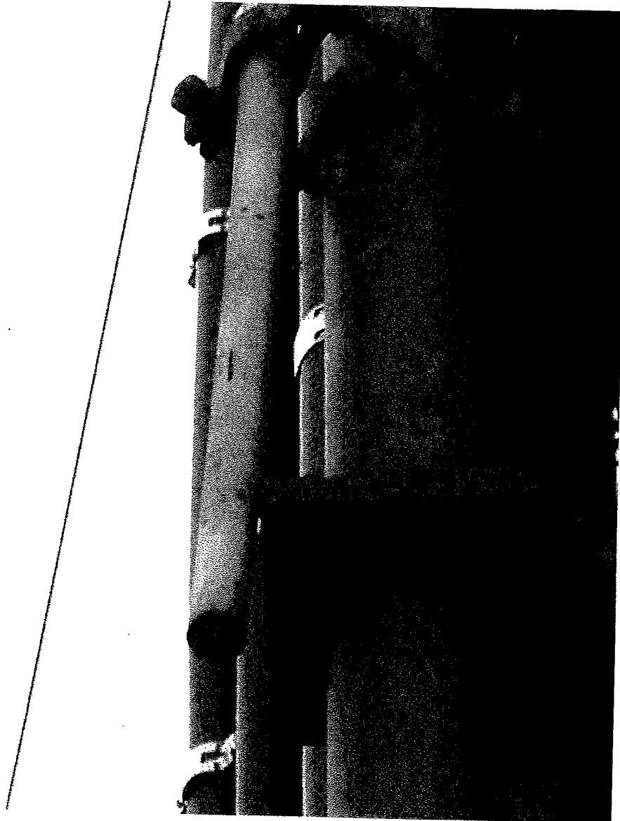
Photo of existing leg reinforcing extending past flange plate.
