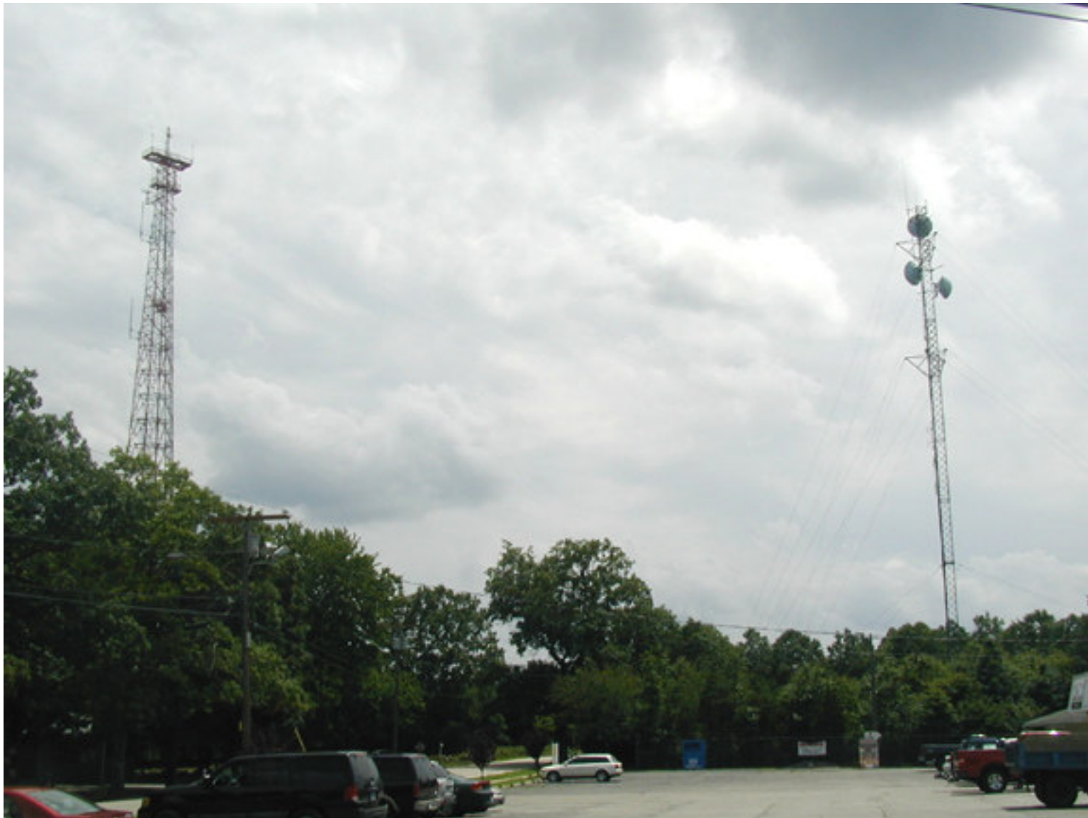
View of two towers – CL&P on right, old AT&T tower on left
