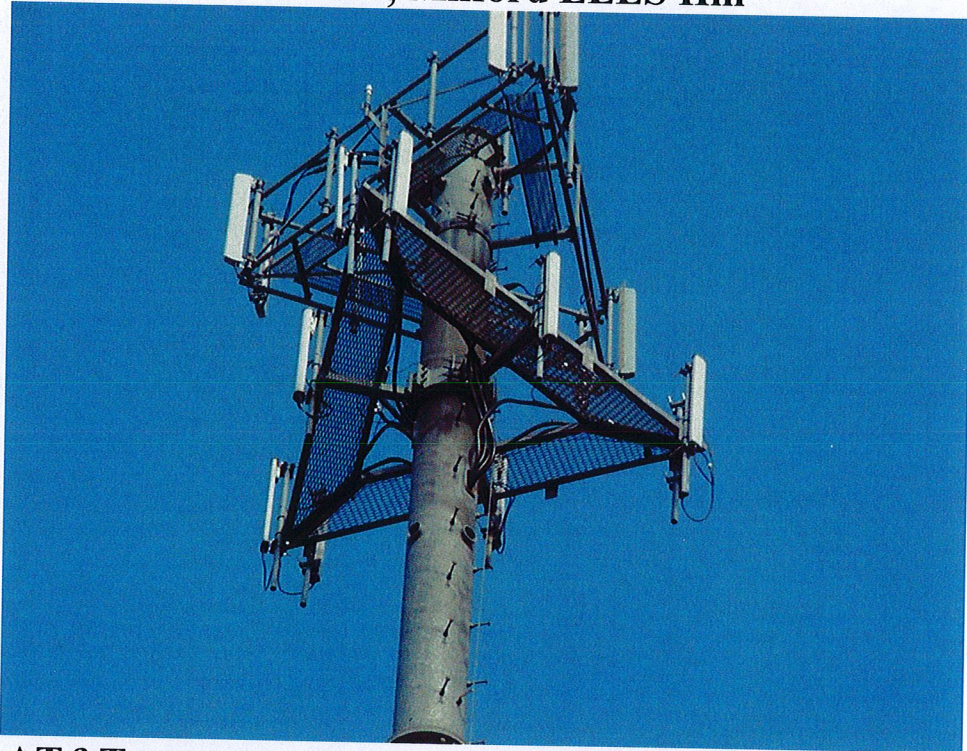
AT&T antenna array before removal (bottom array)
