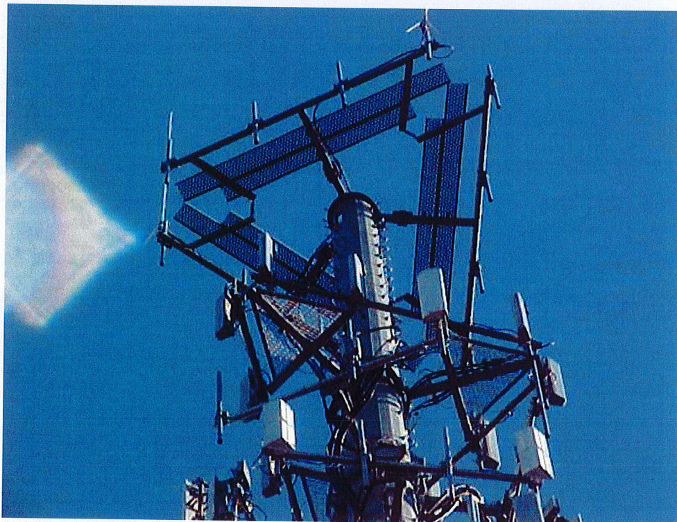
After panels have been removed
