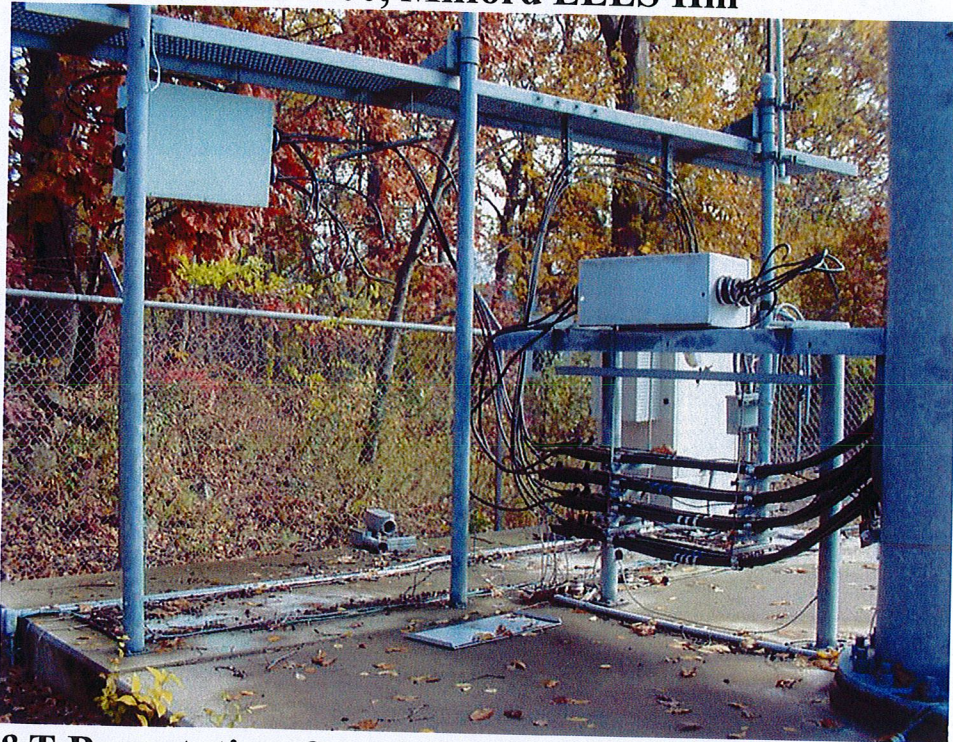
AT&T Base station & associated equipment before removal
