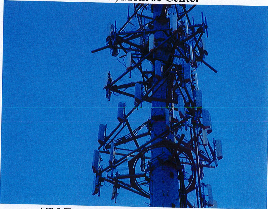
AT&T antenna array before removal
