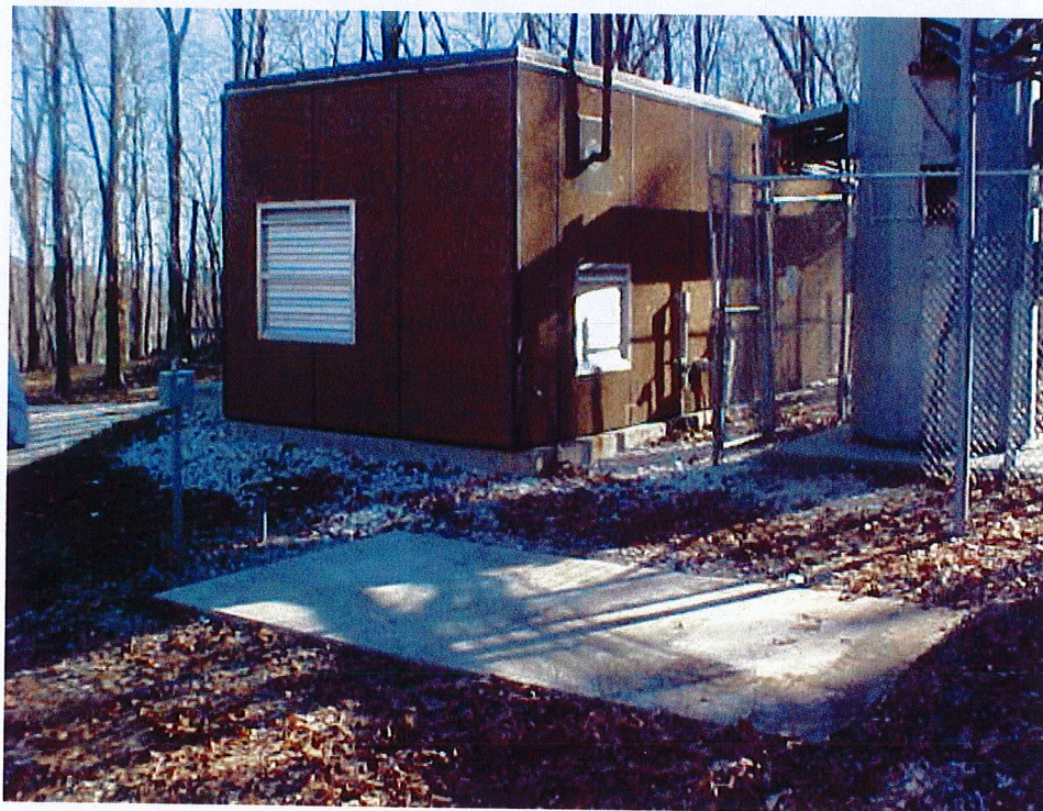
After all base station equipment has been removed
