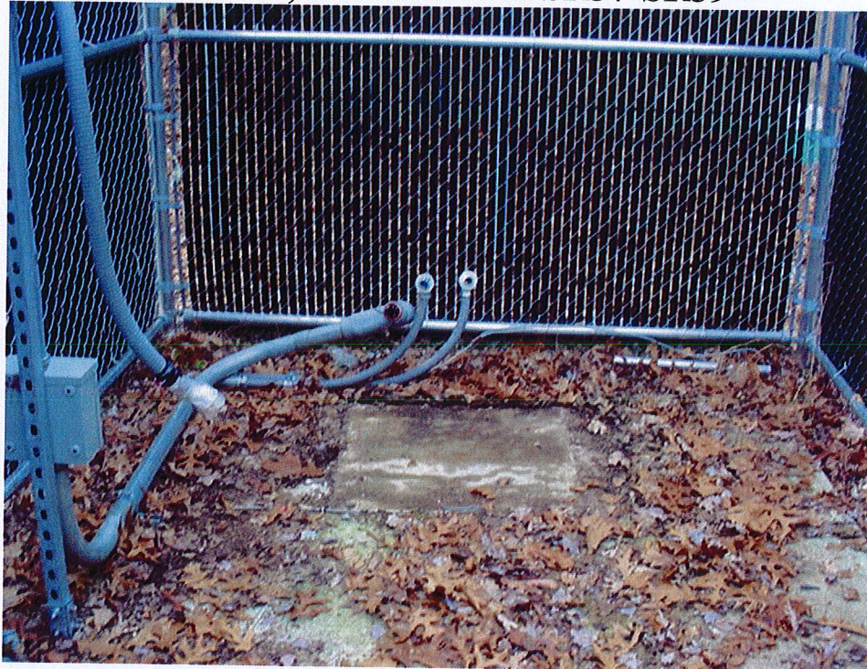
Before all base station components removed
