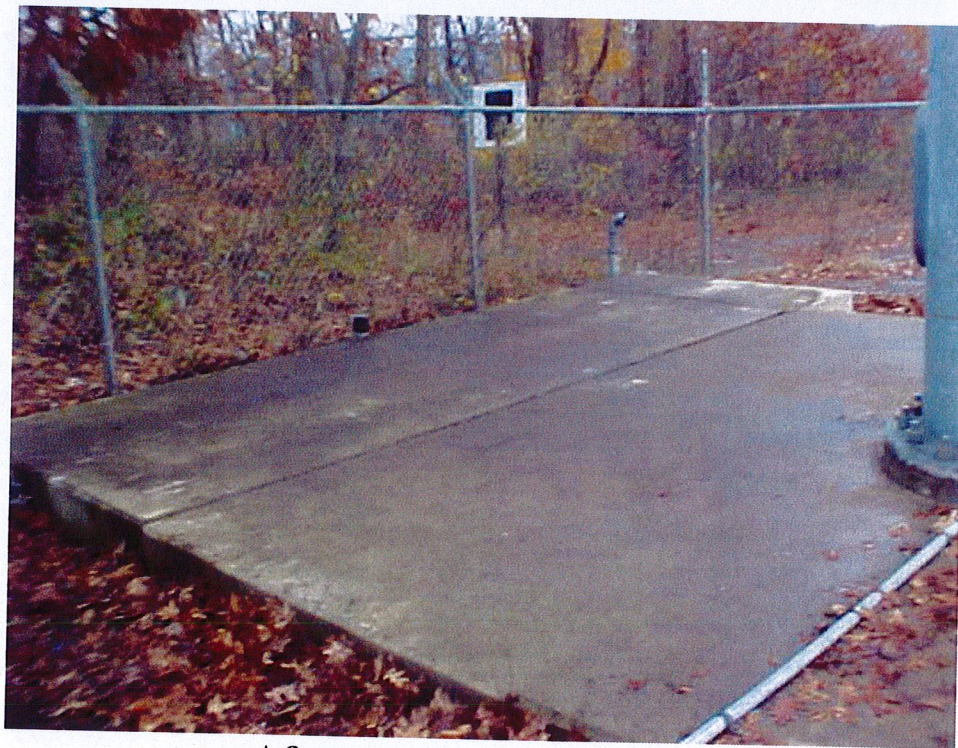
After equipment removal
