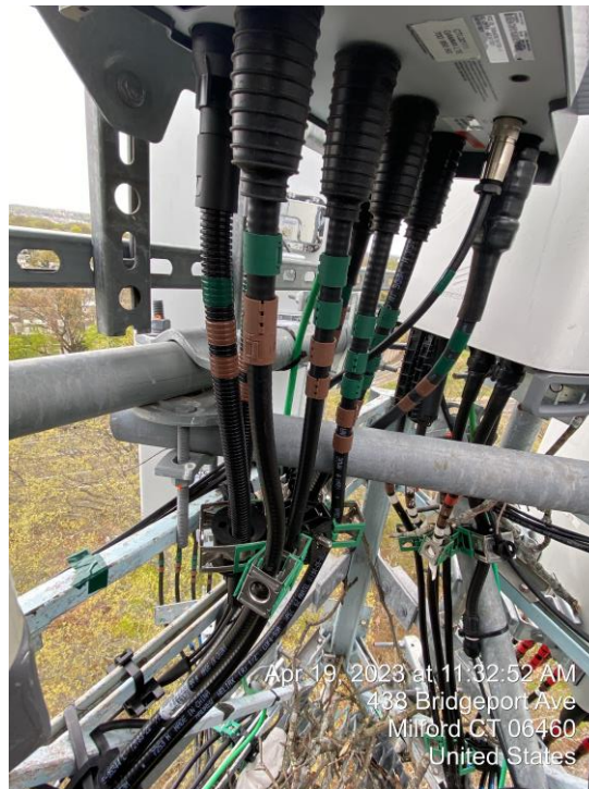
Photo - 4: Installation of proposed remote radio units
