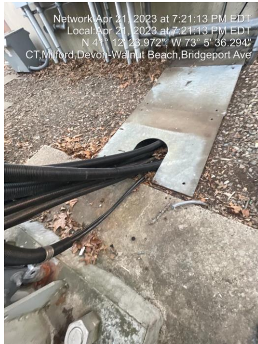
Photo - 5: Installation of proposed cables
