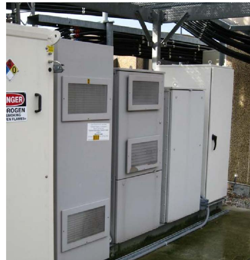
3 EXISTING EQUIPMENT AREA
