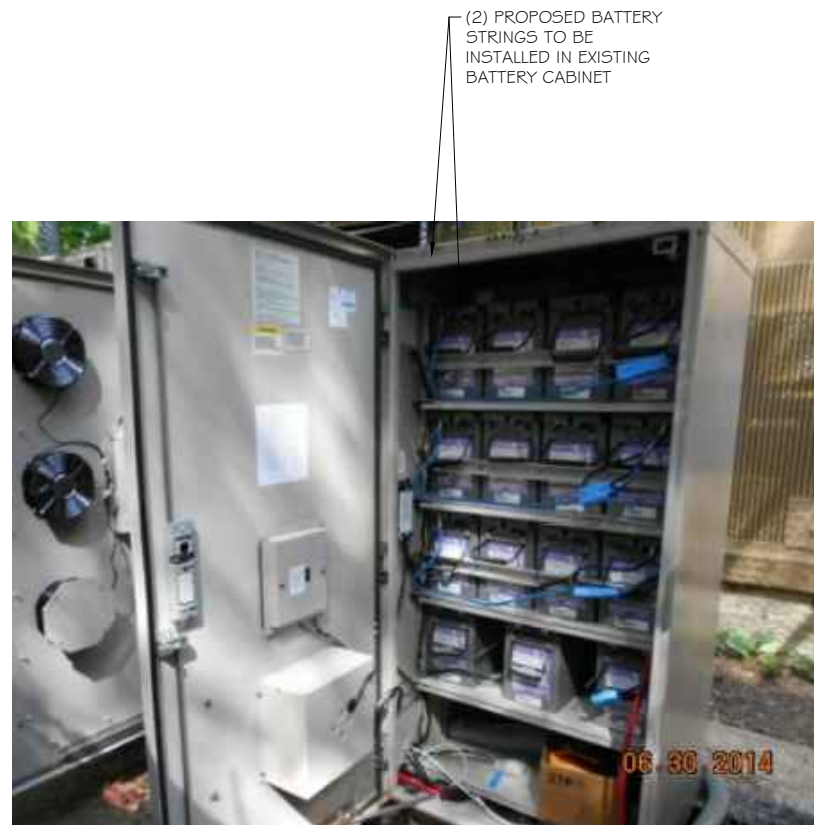
EXISTING BBU CABINET ③ SCALE: NTS
