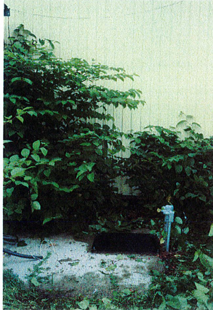
AT&T PAD & ASSOCIATED EQUIPMENT TO BE REMOVED
