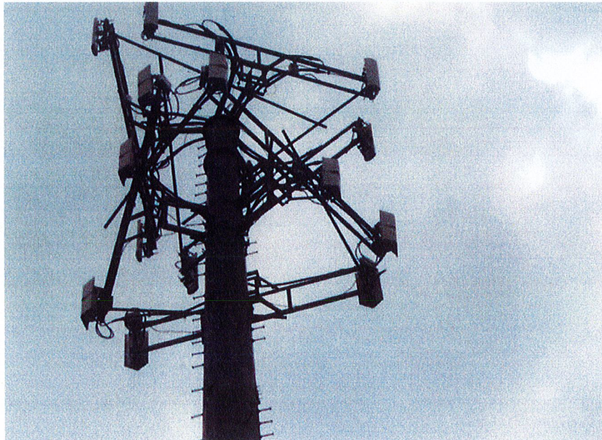
AT&T ARRAY REMOVED AT 165'
