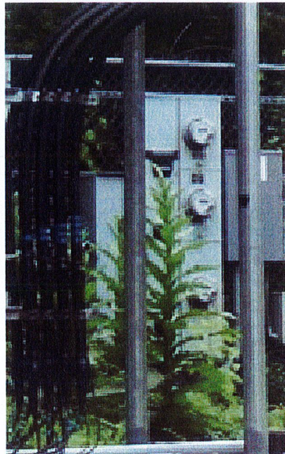
AT&T ELECTRICAL & TELEPHONE TO BE REMOVED
