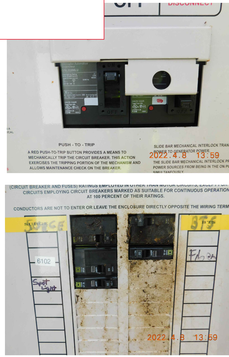
EXISTING POWER PANEL PHOTOS 1 SCALE: NOT TO SCALE E-1
