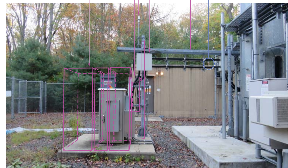
IMAGE SOURCE: PROTERRA 10/21/2017 (VIEW FROM WEST)
