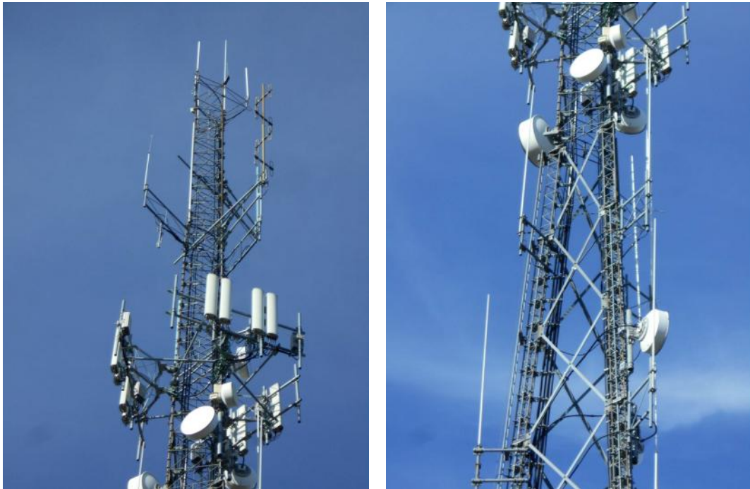
Photos of typical existing equipment and mounts.
