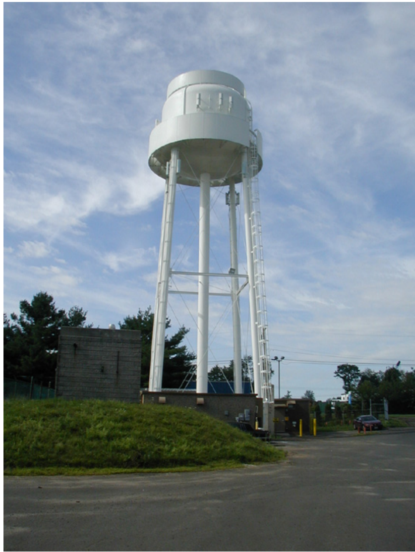
Close up View of Existing Water Tank
