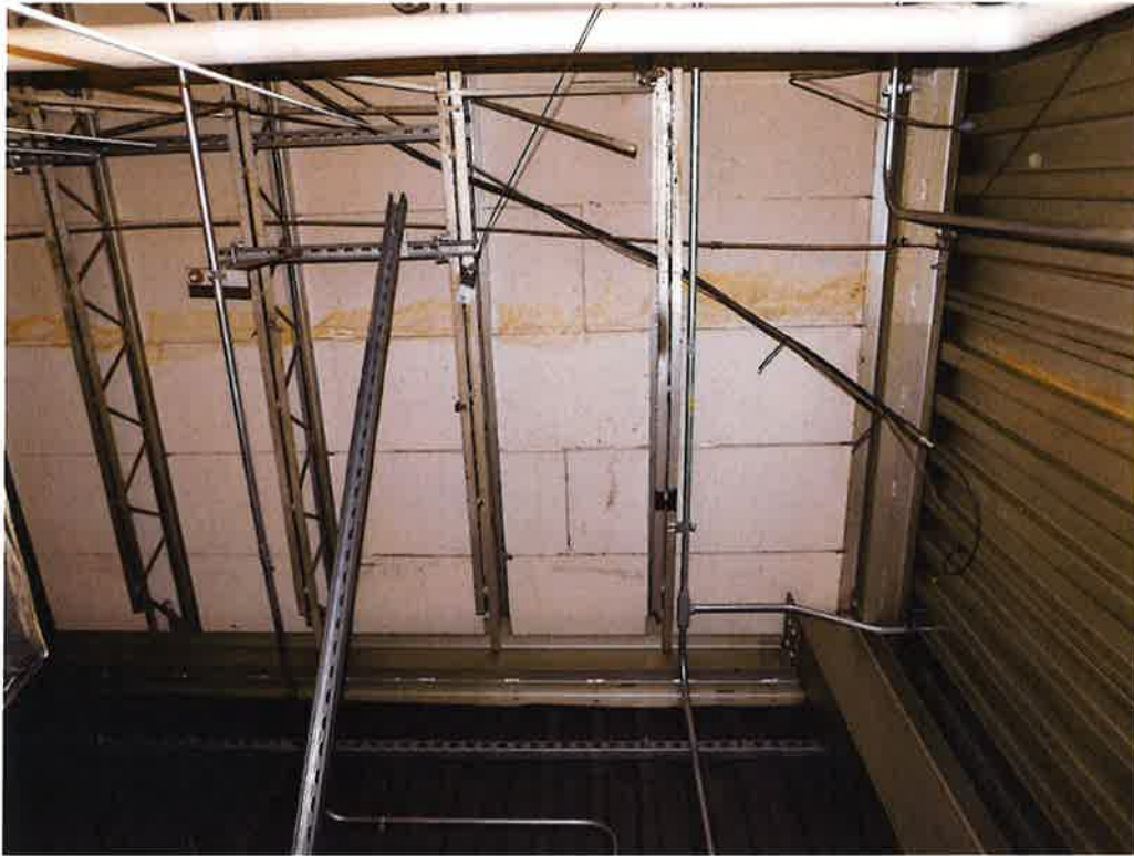
Photo 3: Sample photo illustrating the existing roof framing.
