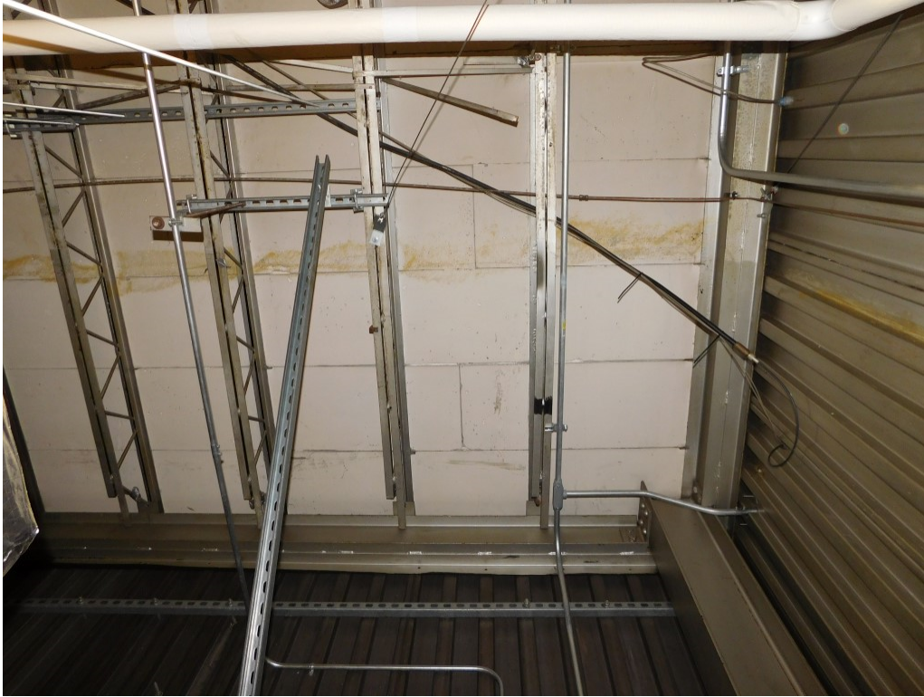
Photo 3: Sample photo illustrating the existing roof framing.
