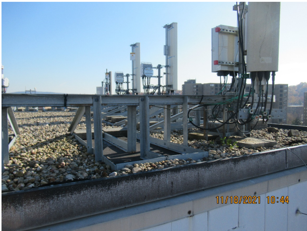
Photo 2: Sample photo illustrating the existing ballast mounts.
