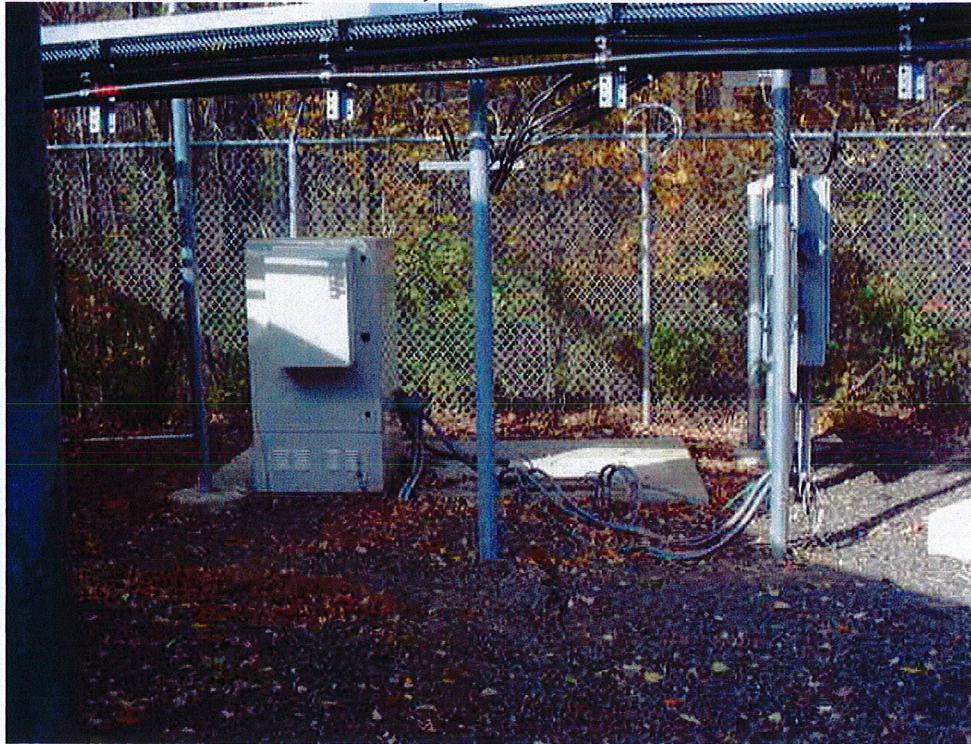
AT&T Base station before removal
