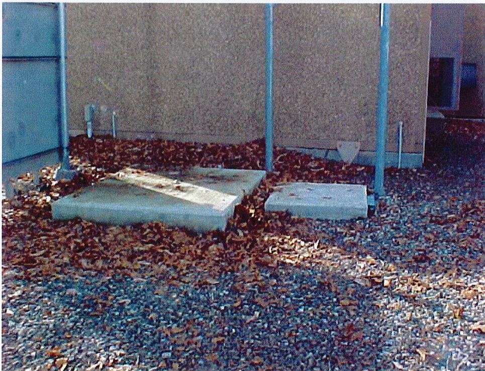
After equipment removal
