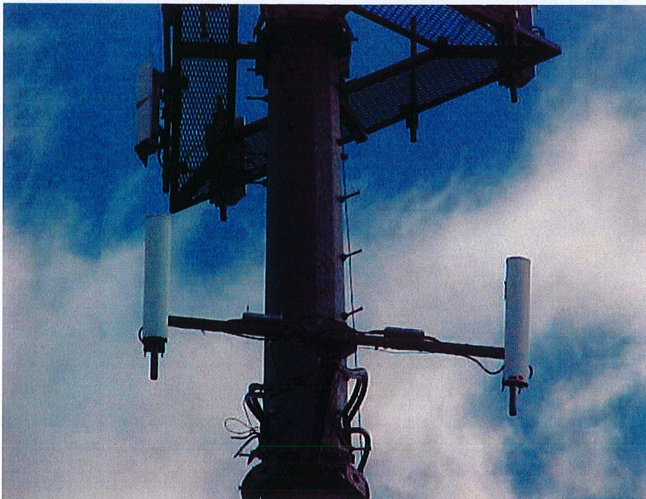
After antenna removal
