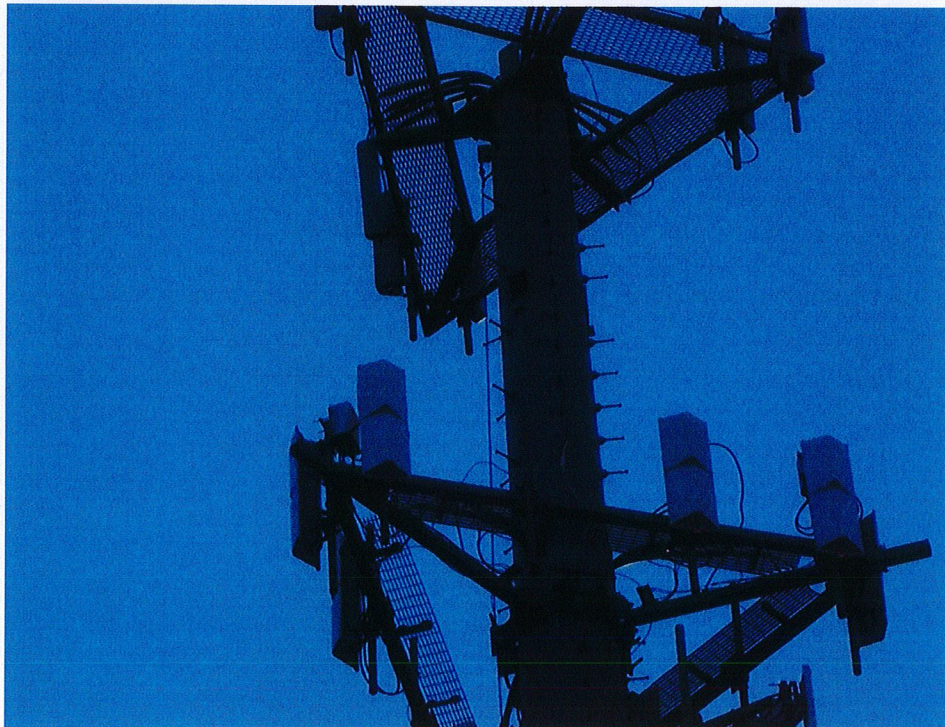
After antenna removal
