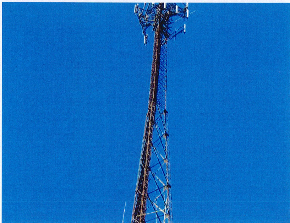
After antenna removal
