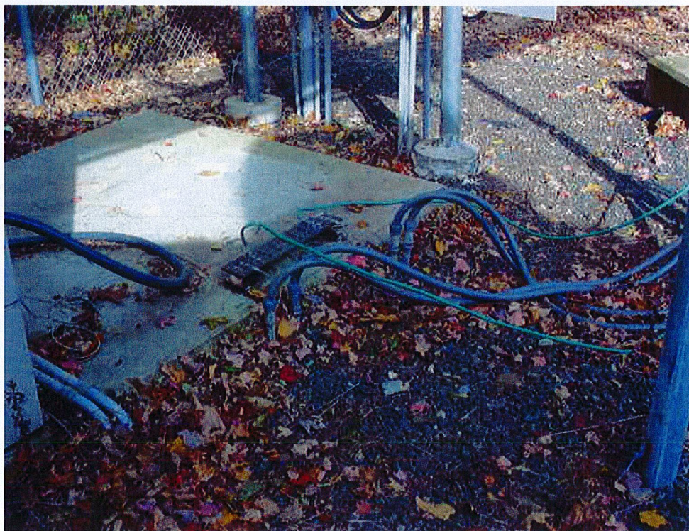
After base station removal
