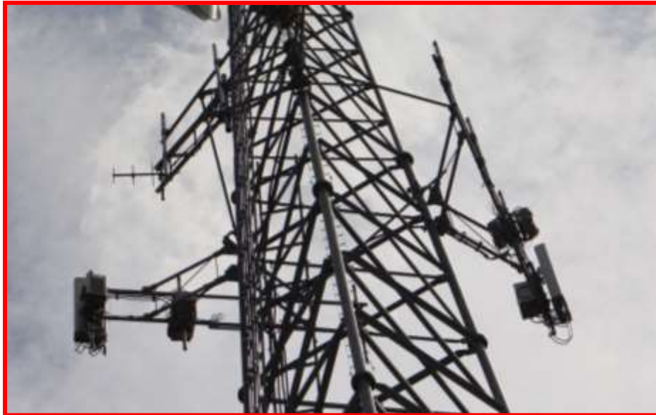
Figure 1 Antenna Mount
