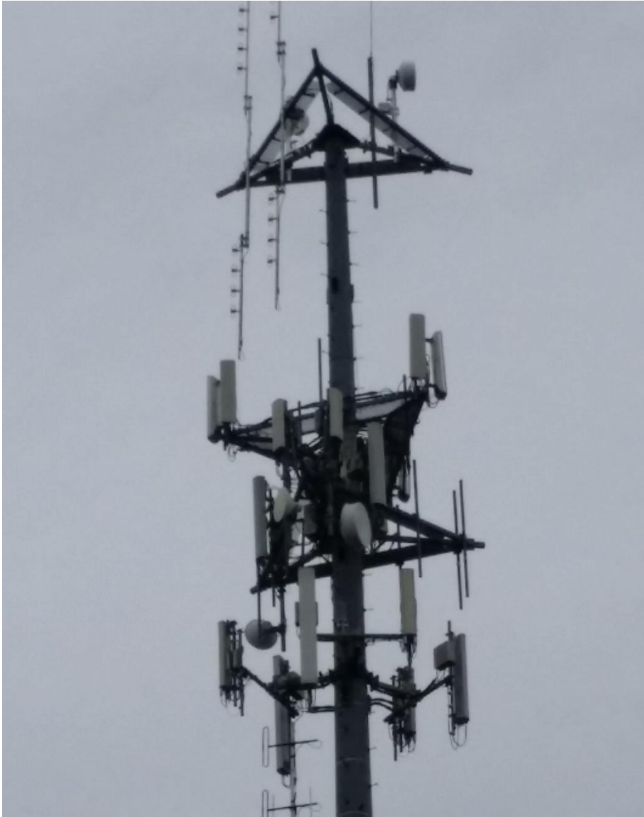
Photo 1: Photo illustrating the Monopole with Appurtenances shown.
