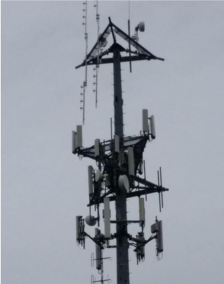
Photo 1: Photo illustrating the Monopole with Appurtenances shown.
