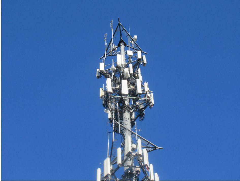
Photo 1: Photo illustrating the Tower with Appurtenances shown.
