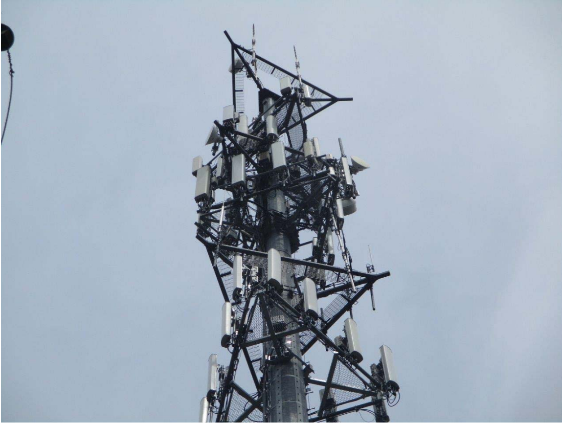
Photo 1: Photo illustrating the Monopole with Appurtenances shown.
