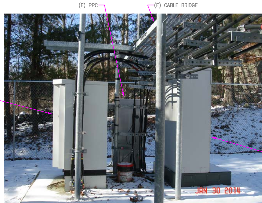
4 EXISTING EQUIPMENT AREA. N.T.S.
