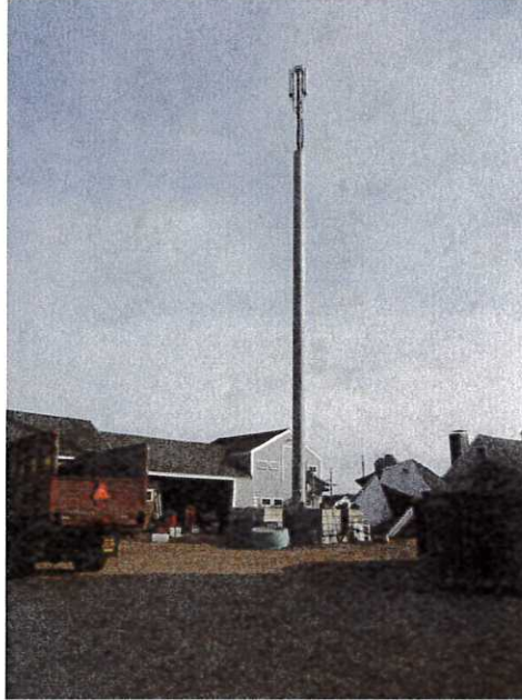
Image of existing \pm 85 -ft tall AT&T temporary uni-pole tower with ballast base frame.
