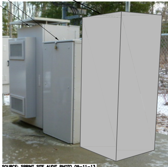
SOURCE: SPRINT SITE AUDIT PHOTO 09-11-13 RAN EQUIPMENT PHOTO DETAIL SCALE: N.T.S.
