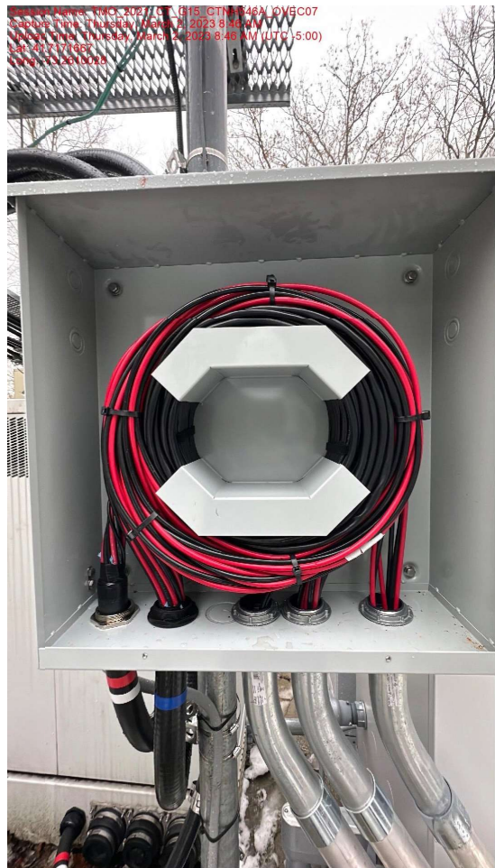
New Slack Box Mounted To Existing Cable Bridge Post
