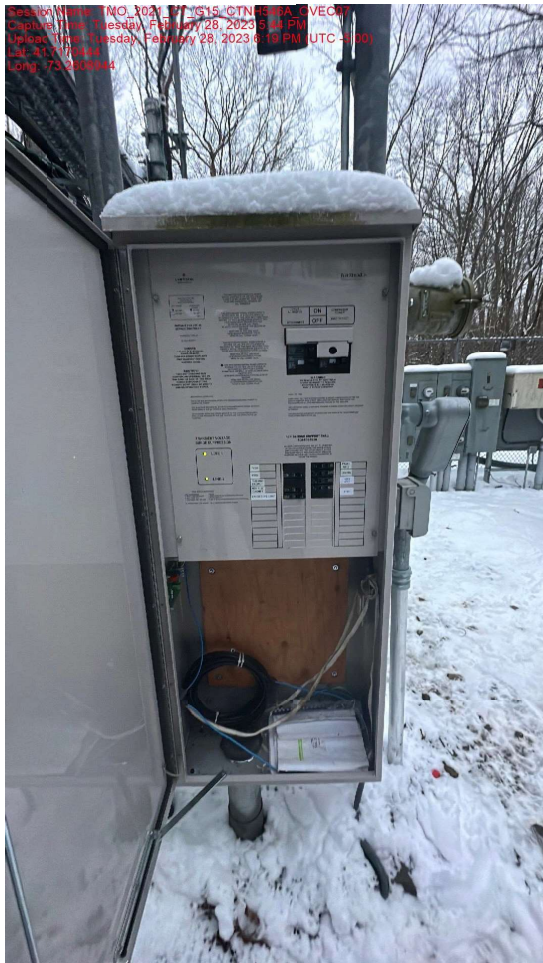
New Equipment Tied Into Existing Electrical Service
