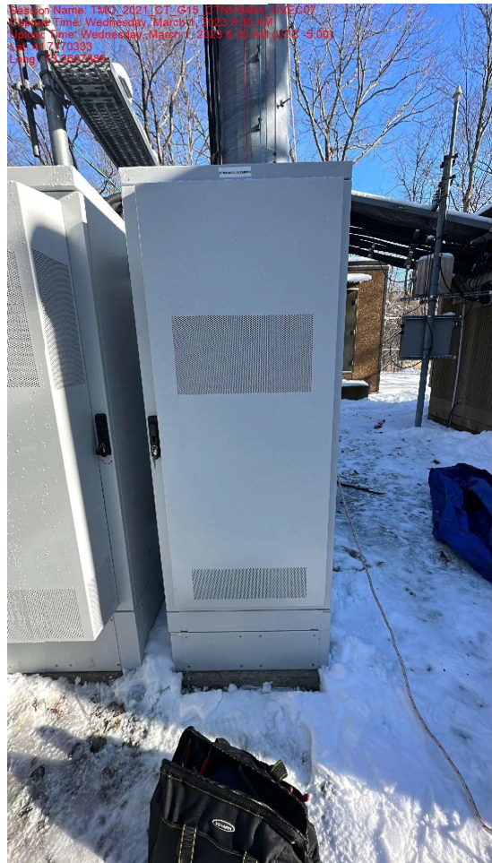
New Battery Cabinet Mounted To New Concrete Pad Extension
