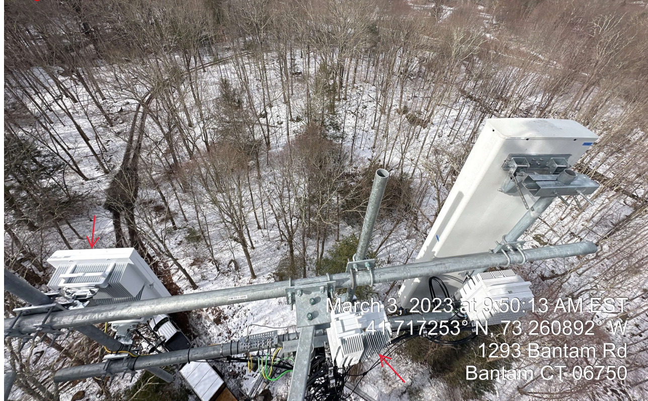
Gamma Sector: (1) New Antenna & (1) New RRH Mounted To Existing Sector Frame
