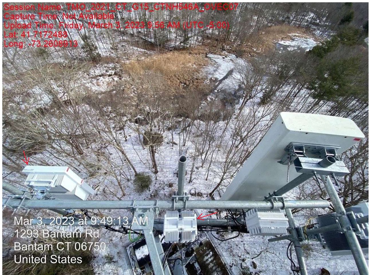
Alpha Sector: (1) New Antenna & (1) New RRH Mounted To Existing Sector Frame
