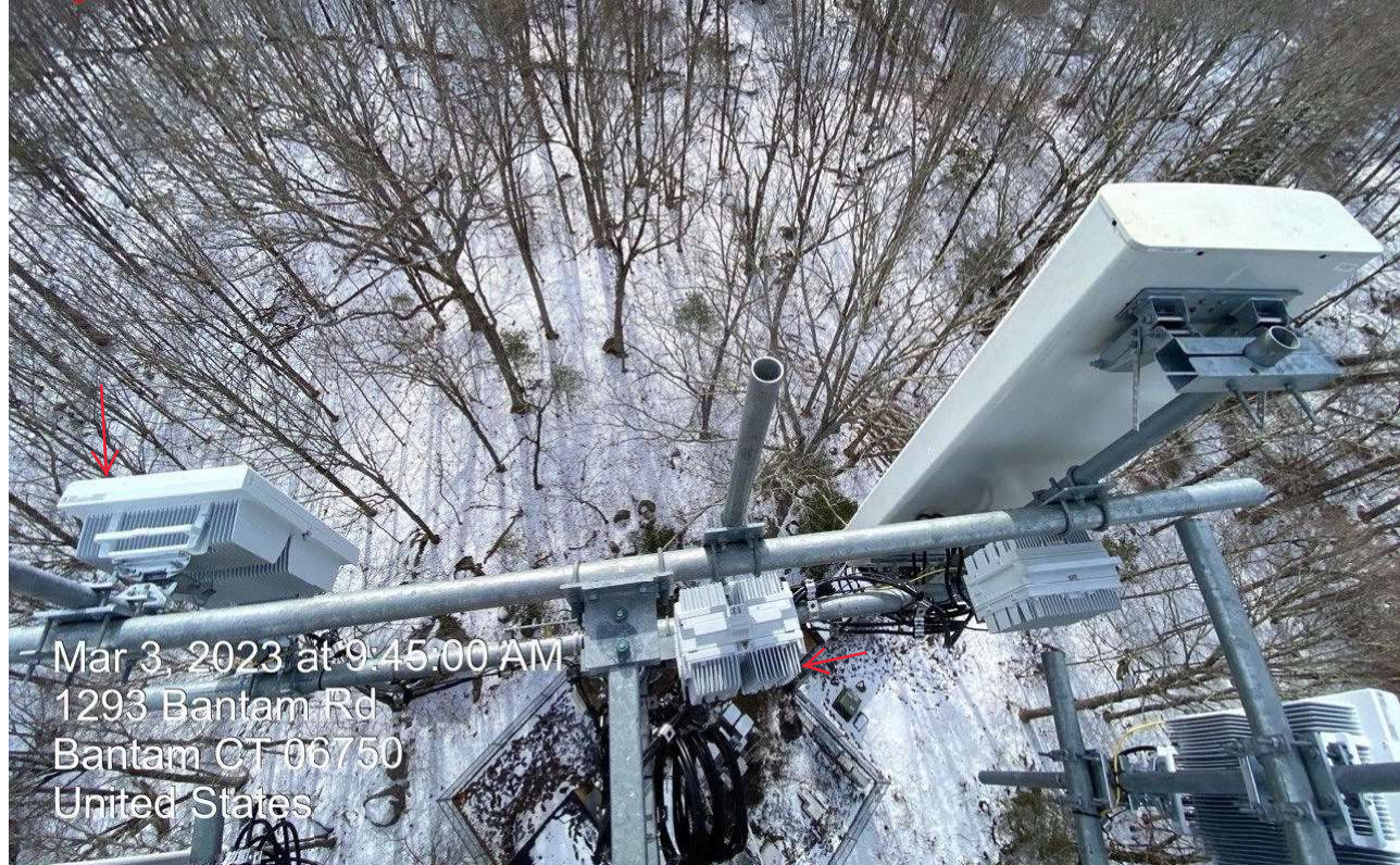
Bate Sector: (1) New Antenna & (1) New RRH Mounted To Existing Sector Frame
