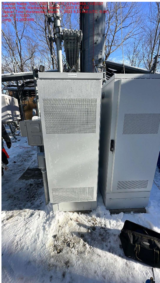
New Equipment Cabinet Mounted To New Concrete Pad Extension
