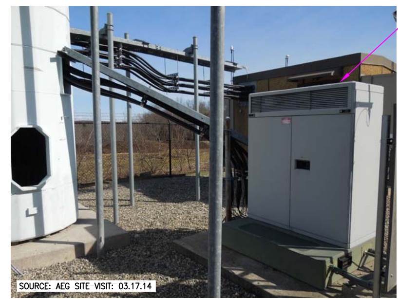
EXISTING EQUIPMENT AREA. N.T.S.
