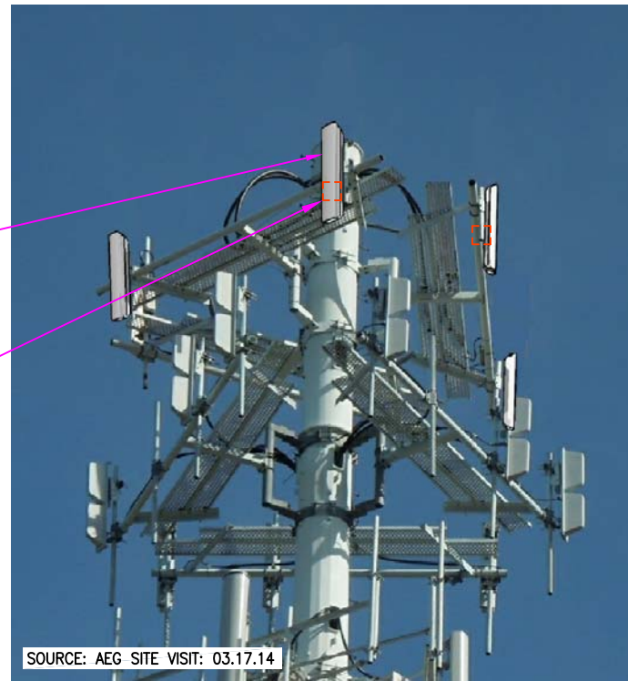
2 A-3 PROPOSED ANTENNA MOUNT TYP. N.T.S.
