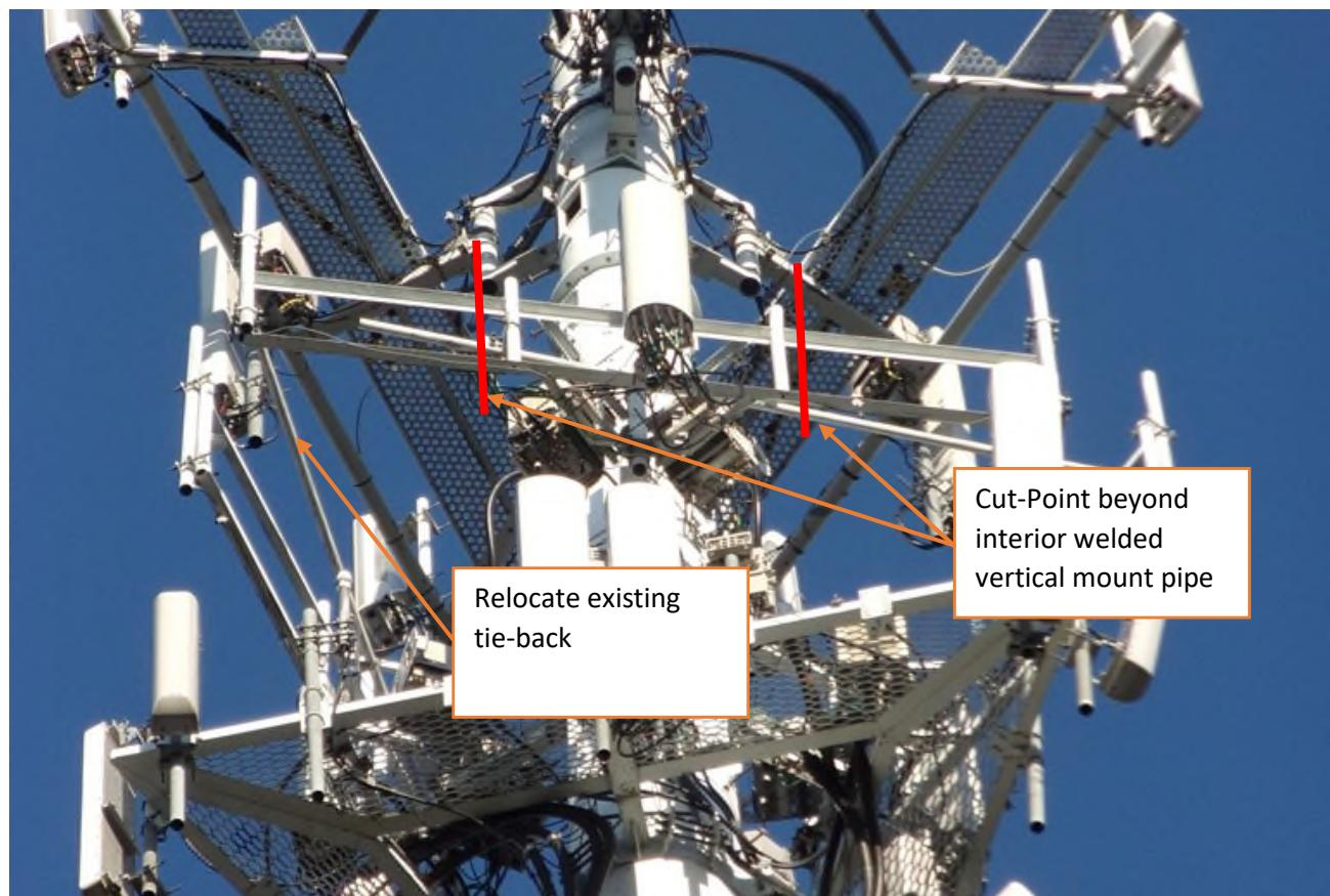
Once the recommended augments are successfully implemented, the **augmented** mount assembly has sufficient capacity to support the loading considered in this analysis pursuant to the listed standards.
