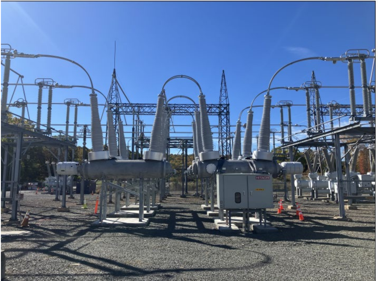
Newly Installed Circuit Breaker
