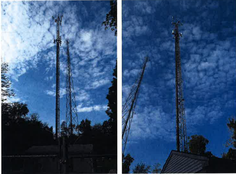
Overview photos of 190' guyed tower.
