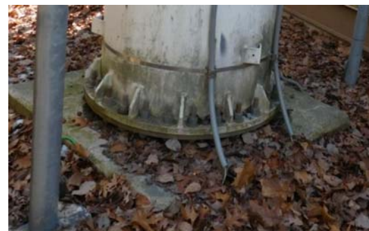
MONOPOLE TOWER BASE FOUNDATION PHOTO
