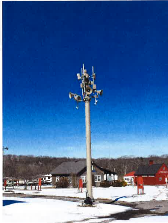
Overview image of ±30-ft steel monopole tower.
