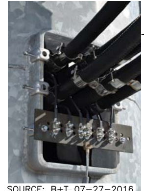
2A FEEDLINE PHOTO DETAIL @ TOWER BASE SCALE: N.T.S.
