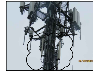
MODIFICATION INTERFERENCE EL: 69'-0"±
