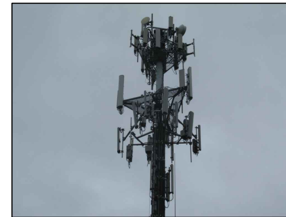
POSSIBLE MODIFICATION INTERFERENCE EL: 75'-0"± TO 87'-0"±
