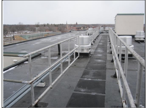
10. Sprint/Clearwire Sector A transmission direction
