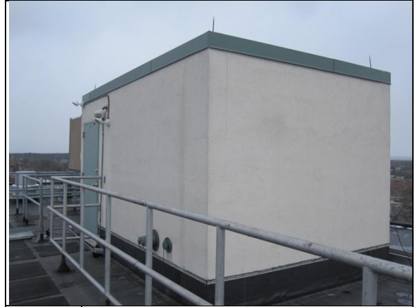
28. Penthouse with roof access
