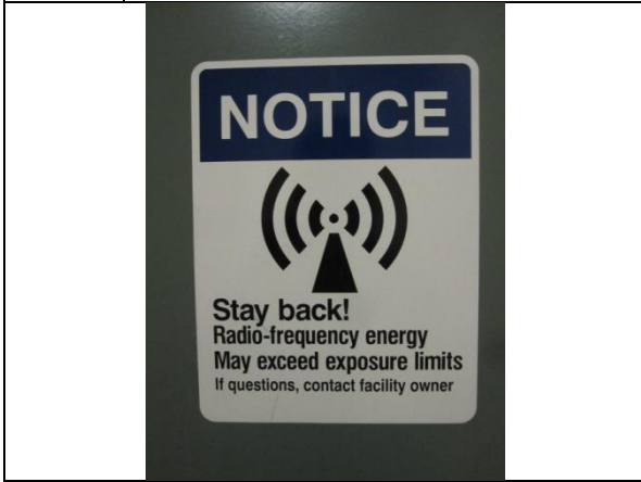
3. Roof access door existing signage detail
