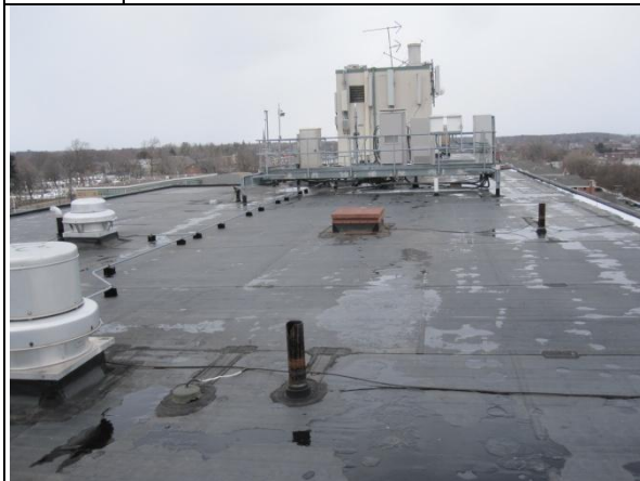
27. Roof overview looking North towards Sprint Sector B
