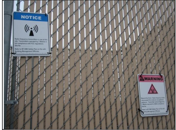
4. Existing signage on T-Mobile equipment compound fence_1
