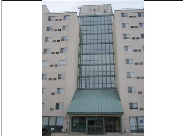
13. Building aspect looking towards Sprint/Clearwire Sector C
