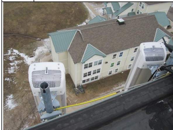
15. T-Mobile Sector A – roof view
