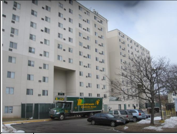
31. Building aspect looking
