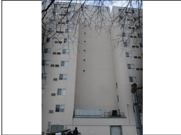
19. T-Mobile Sector B - ground view 1
