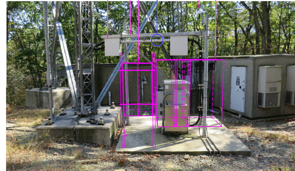
IMAGE SOURCE: PROTERRA 10/19/2017 (VIEW FROM NORTHWEST)
