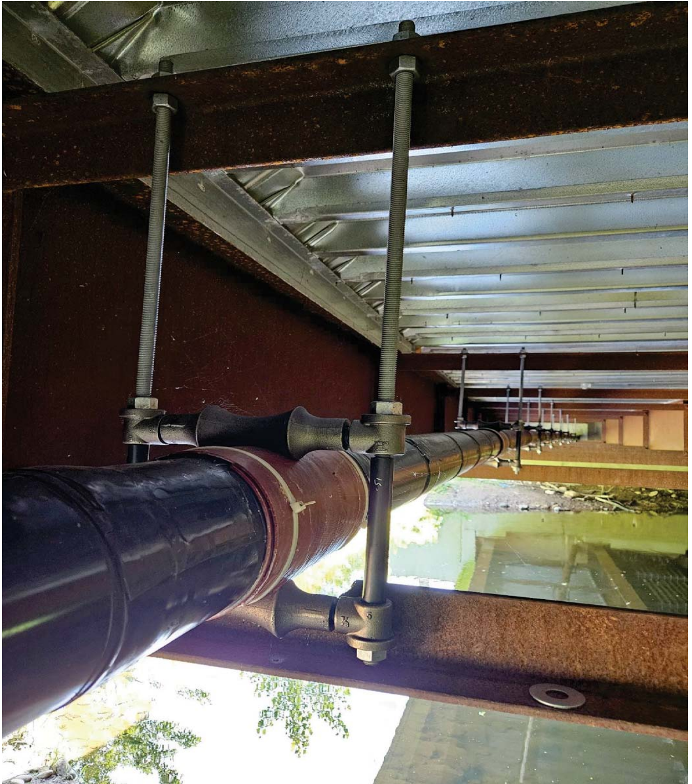
Photo 2: New Hanger Unit
