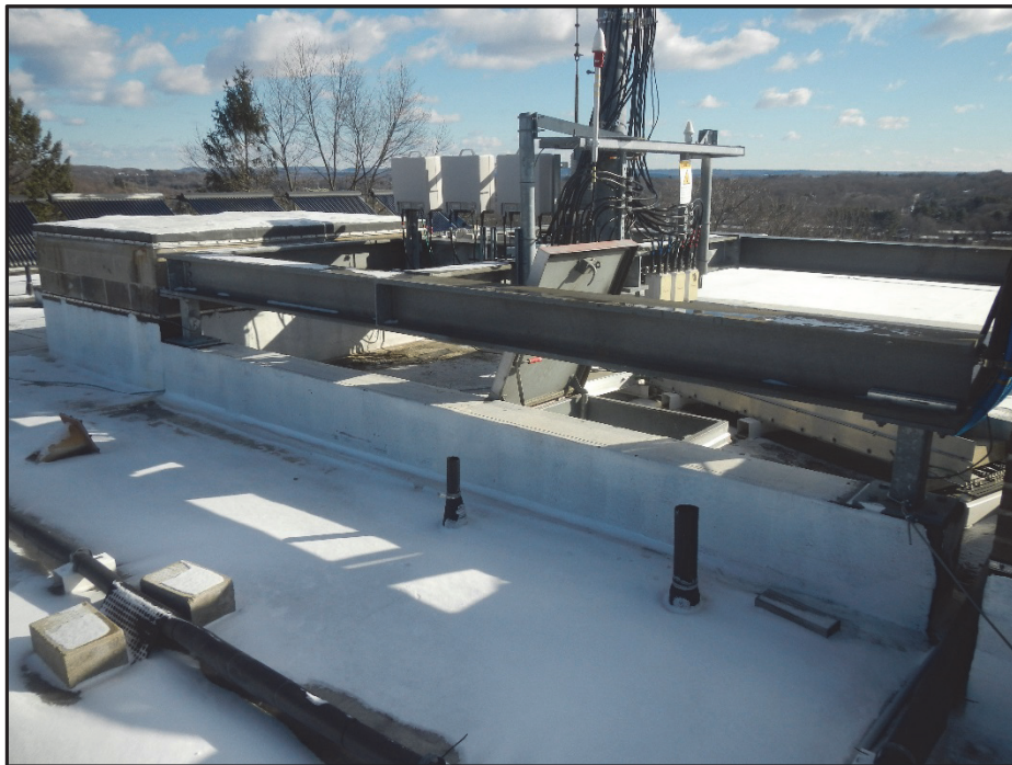
EXISTING STEEL PLATFORM ANCHORED TO ROOF STRUCTURE
