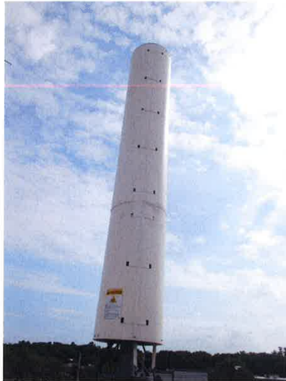
Photo 1: Sample photo illustrating the existing FRP enclosure to be removed.
