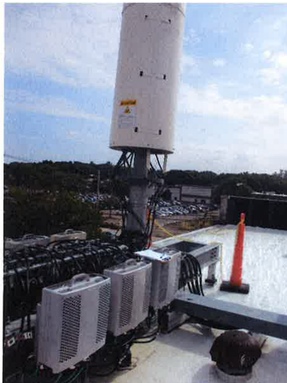
Photo 2: Sample photo illustrating the existing RRH's.
