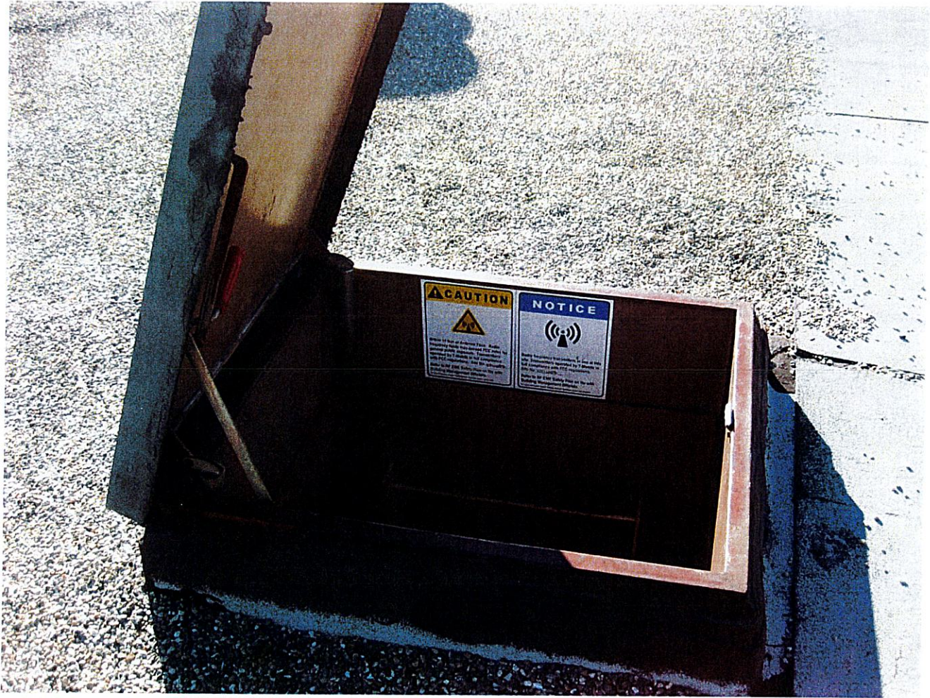
Figure 3: Roof Access Door
