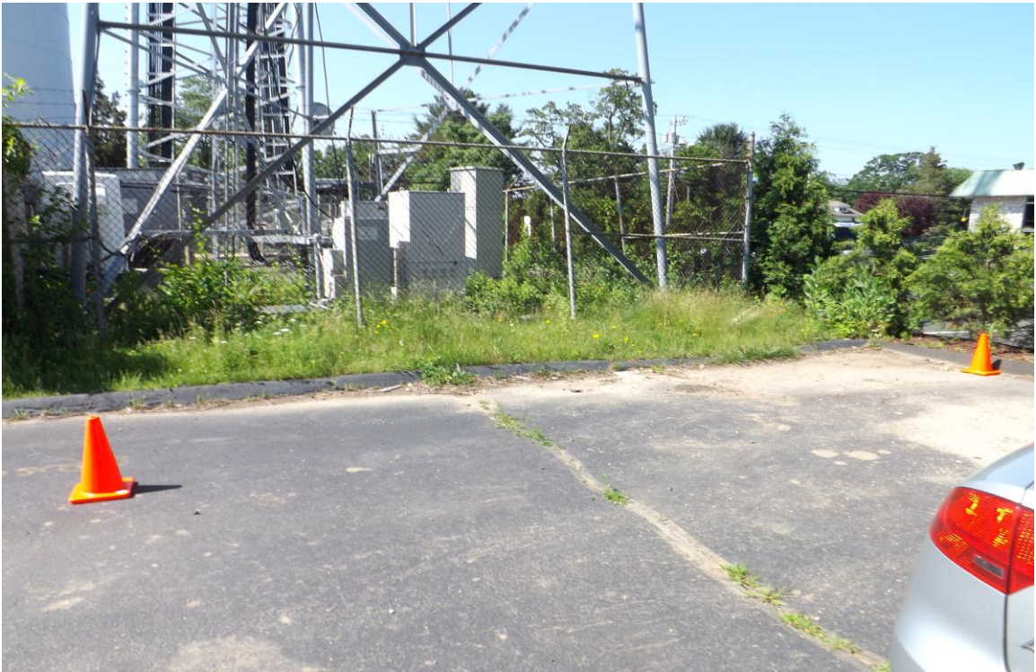
The corners of the proposed expanded compound are marked with orange cones.
