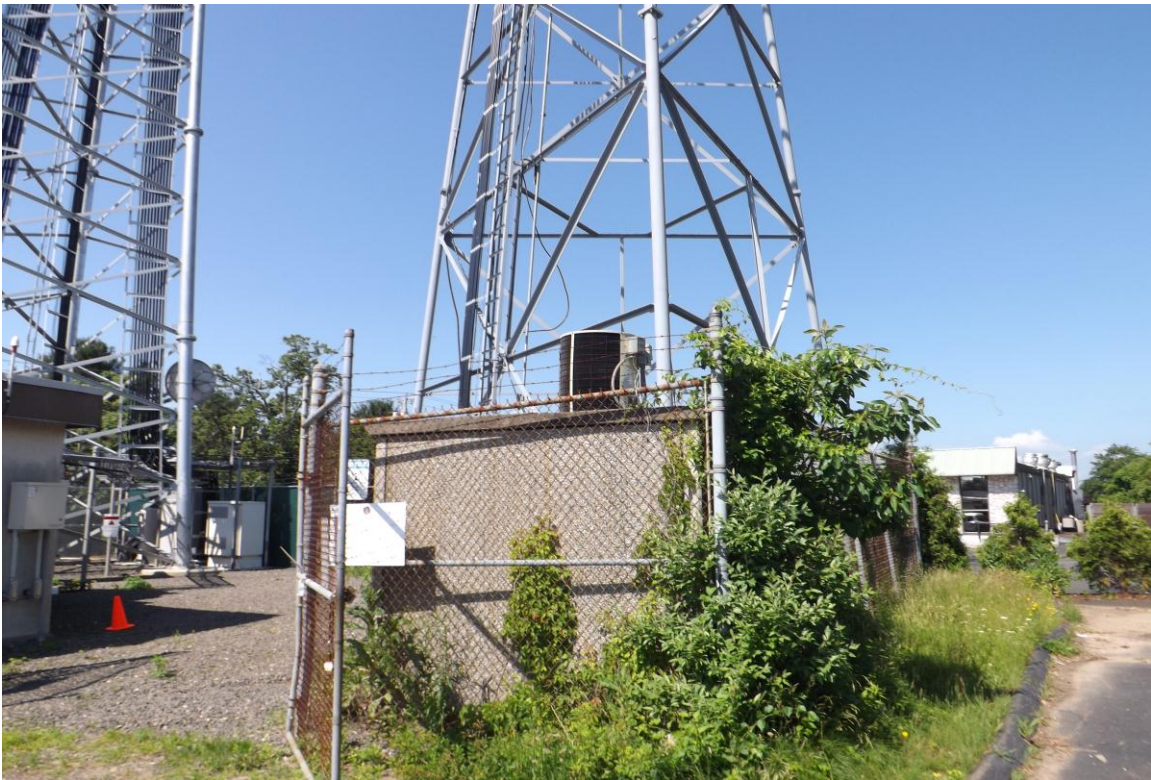
Existing 88-foot lattice tower proposed to be removed and replaced with a 150-foot monopole.
