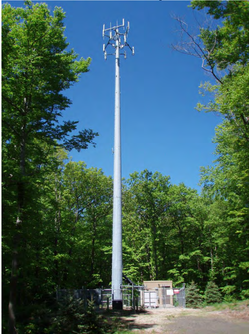
View of Tower and Compound
