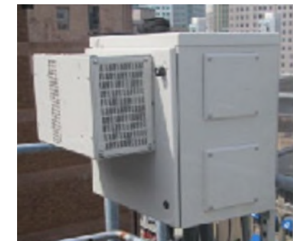
EMERSON NETXTEND COMPACT 2416 CABINET ENCLOSURE: ALUMINUM DIMENSIONS (HxWxD): 24" X 24" X 25.25" WEIGHT: 64LBS (EXCLUDES EQUIPMENT) WEATHER TIGHTNESS: NEMA TYPE 3R
