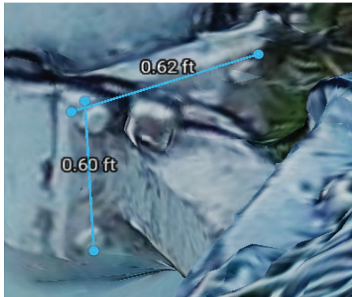
Picture #12 - Flange Plate Dimensions
