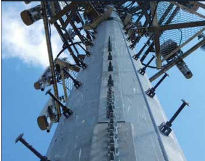
PH#03 Installation of Modification – Installed Flat Plate Reinforcement (119.25'-129.25')
