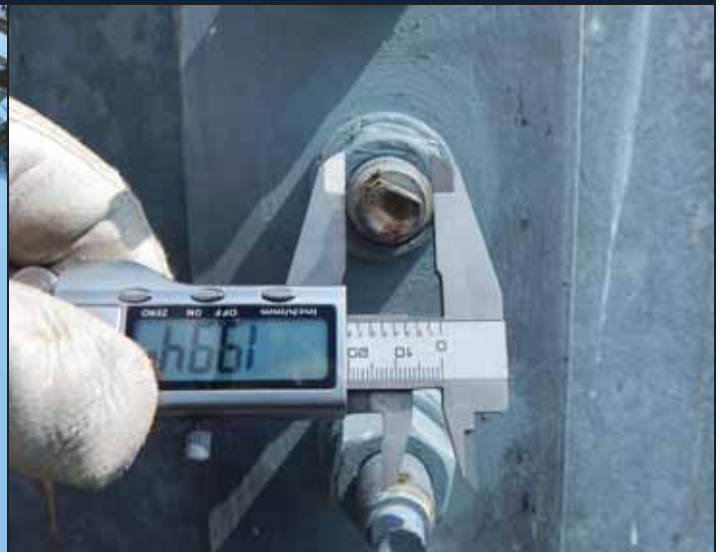
PH#04 Installation of Modification – Blind Bolt Diameter (119.25'-129.25')
