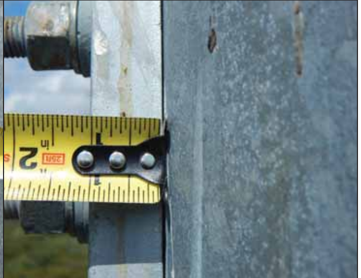
PH#08 Installation of Modification – Maximum Intermediate Bolt Spacing (119.25'-129.25')
