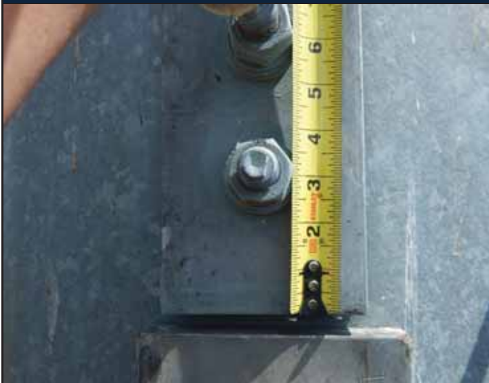
PH#07 Installation of Modification – Flat Plate Edge Distance and Bolt Spacing (119.25'-129.25')
