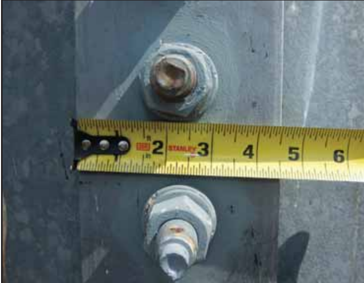
PH#07 Installation of Modification – Flat Plate Edge Distance and Bolt Spacing (119.25'-129.25')
