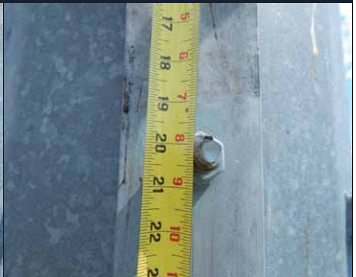
PH#08 Installation of Modification – Maximum Intermediate Bolt Spacing (119.25'-129.25')
