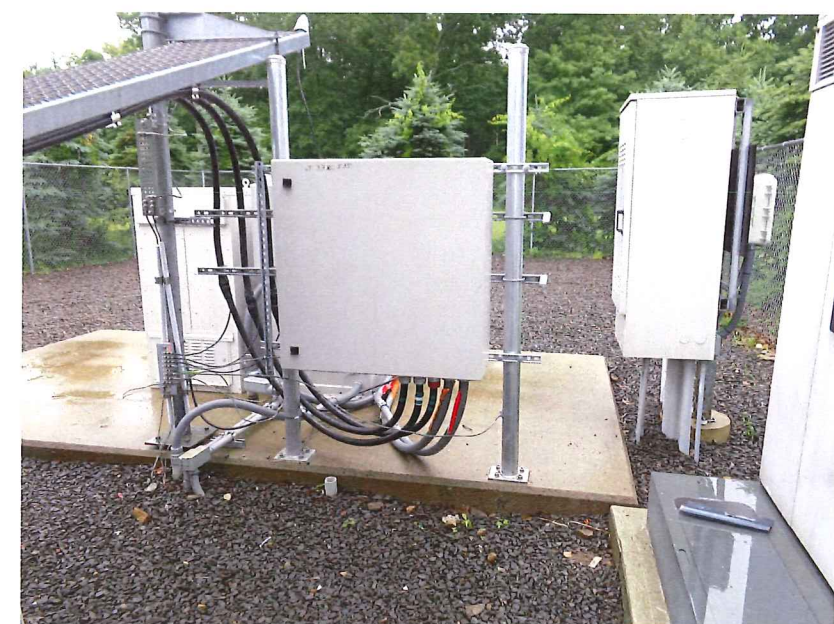
4 EXIST FIBER DISTRIBUTION BOX SCALE: NTS
