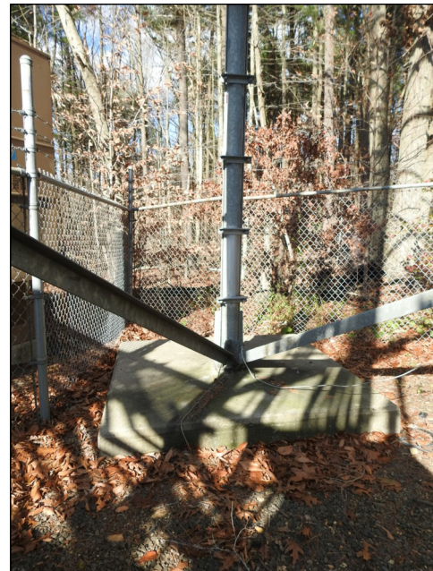
TOWER BASE/FOUNDATION PHOTO
